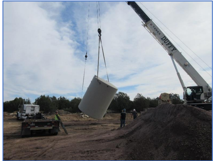
Figure 3: Installation of oil and water tanks
