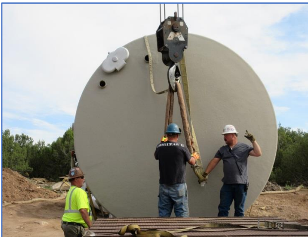
Figure 4: Installation of oil and water tanks
