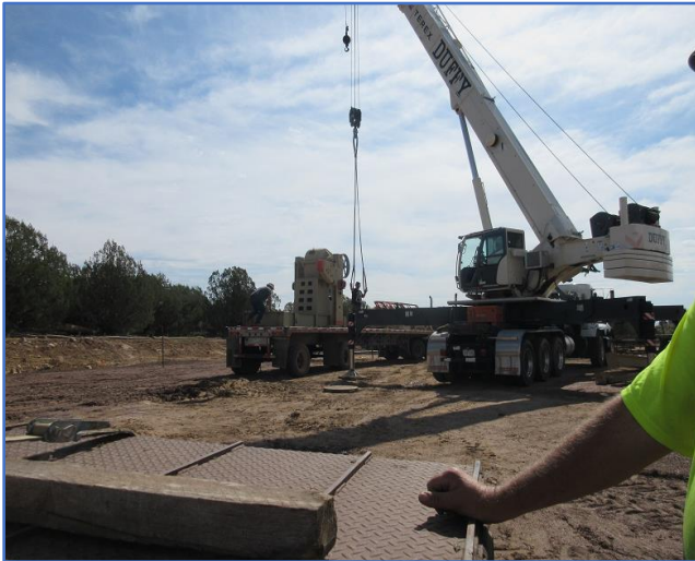
Figure 2: Installation of Pump-Jack
