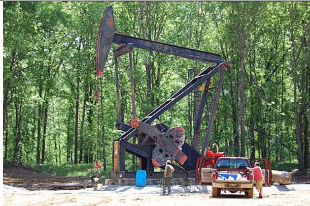
Pumpjack is Installed
