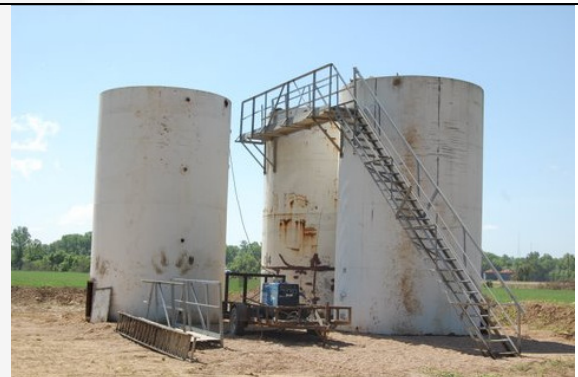
Tank Battery Prior to Completion
