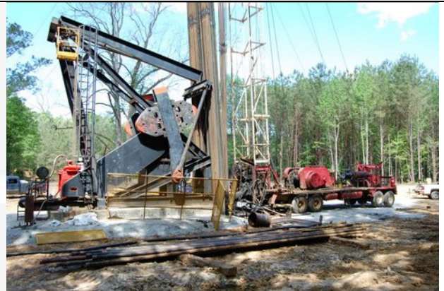
Armstrong Sand Perforation Work
