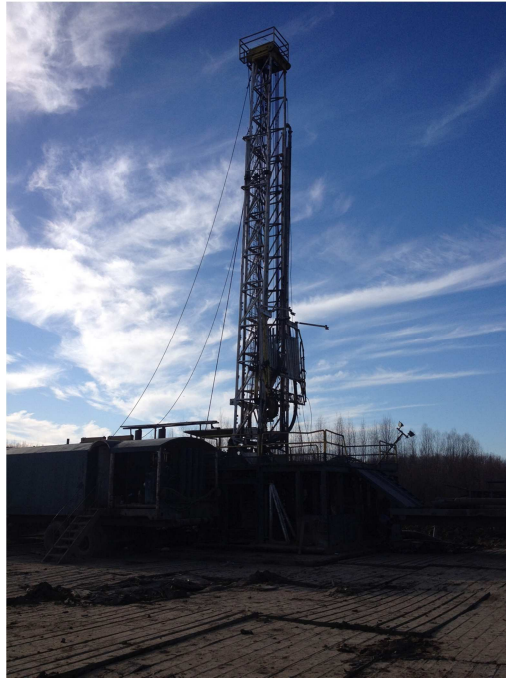
Bourke #5 Drilling Rig
