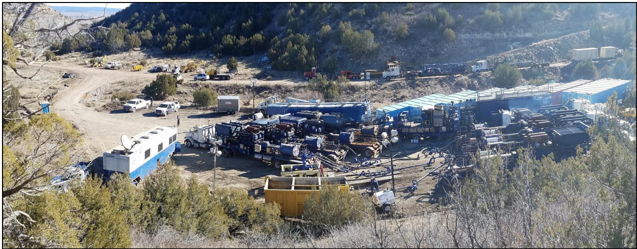
Figure 1: Fracking and completion operations underway
