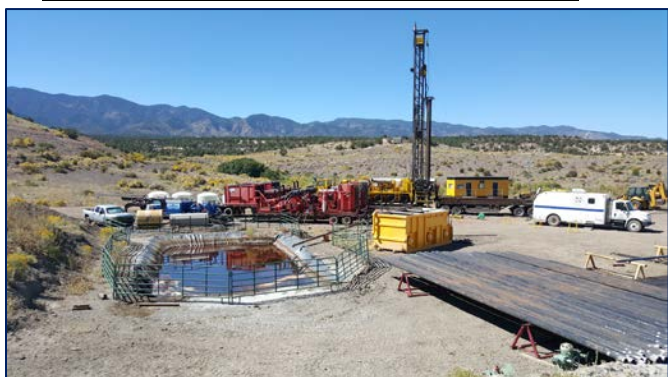
Drilling underway on the Columbus #1 well
