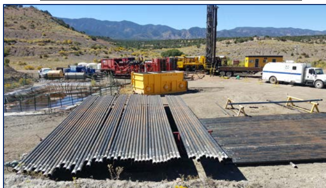
Production casing on location for the Columbus #1 well
