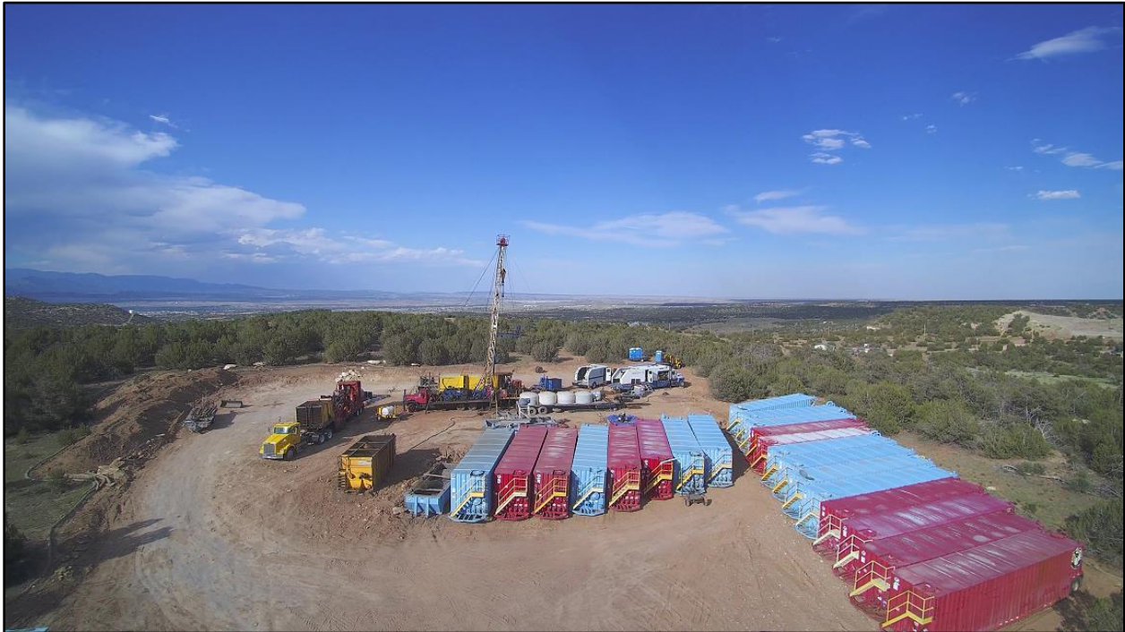
Figure 1: Completion operations on the Amerigo Vespucci #1 well.
