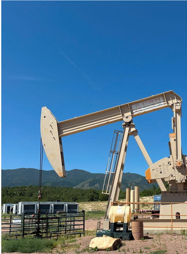
Pathfinder Well with Modular Data Centre in Background
