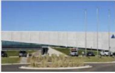
Perimeter Technology Oklahoma City 22,000 SF
