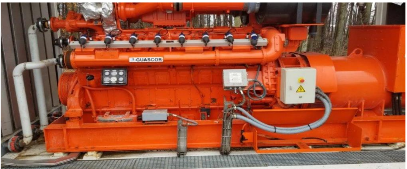
Images 1-4: AXP's Colorado lease ready for the commencement of earthworks (1 & 2) and power generator units being loaded for transportation to site (3 & 4)
