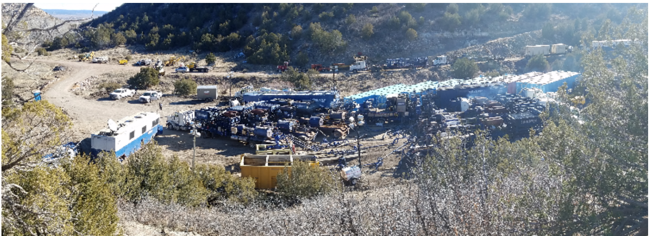
Image 1: Completion of the JW Powell well in 2019
