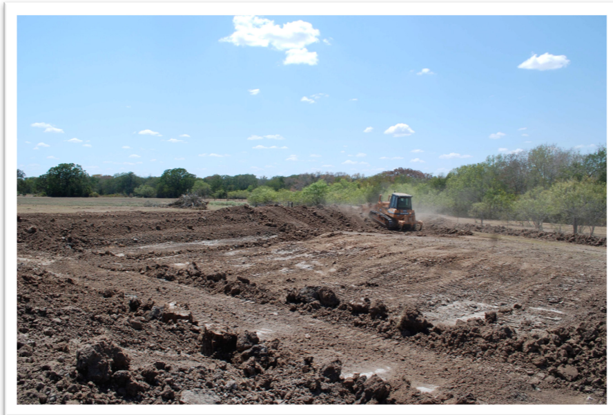
Krueger #1 – Pits being dug out
