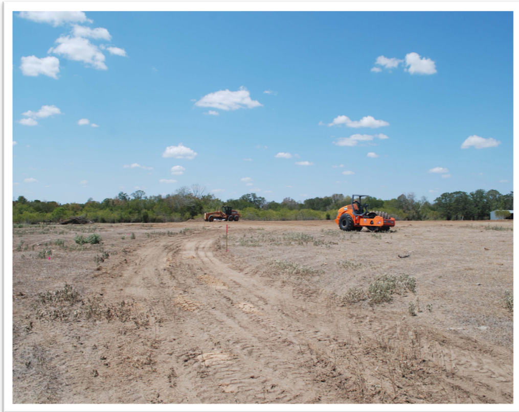
Krueger #1 – Drill site Location (Pad Work)
