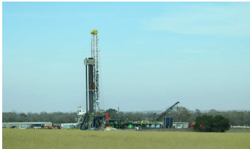
An Image of the Shamrock #1 Rig Spudding the Mississippi #4 Well
