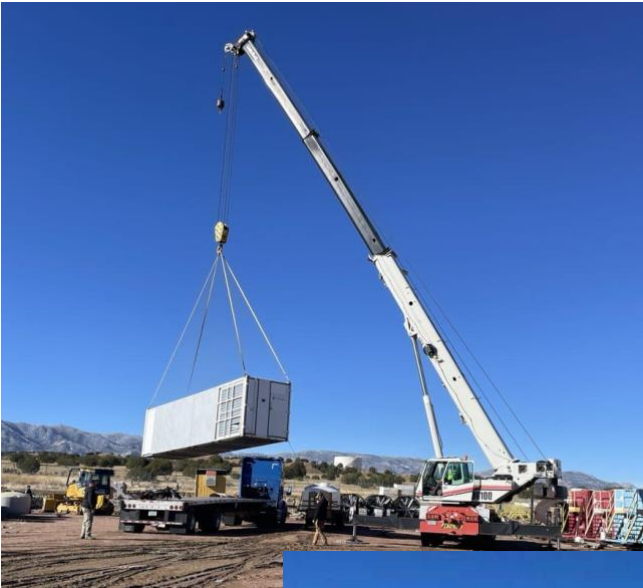
MDCs BEING UNLOADED IN COLORADO
