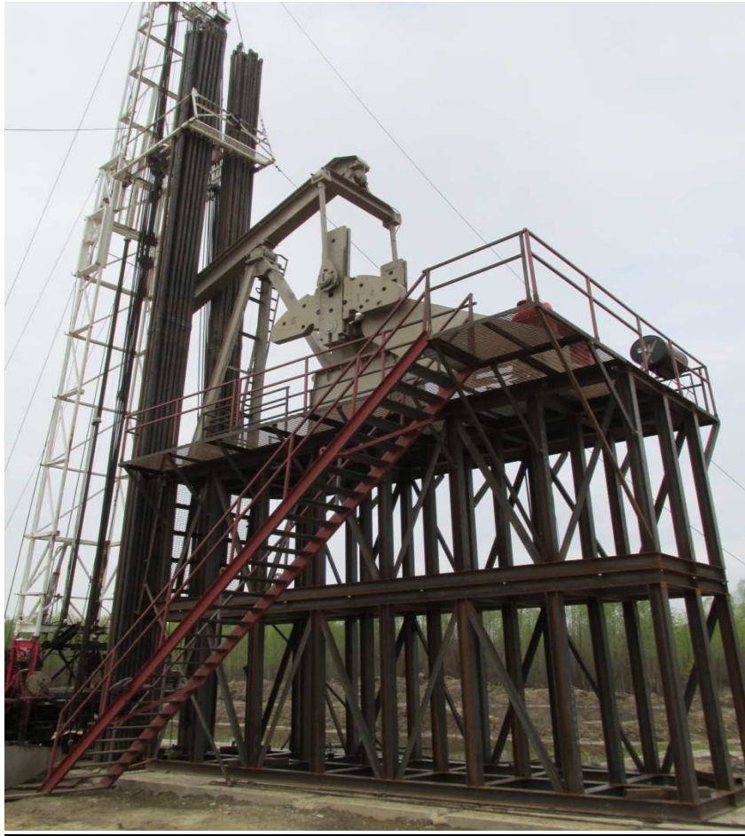
Image of MS#4 Elevated Pump Structure & Rig
