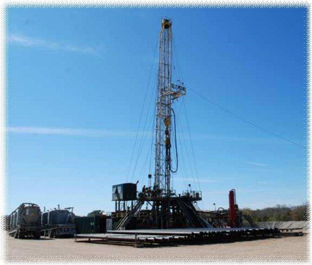
Drilling Rig at Krueger Unit #1 Well
