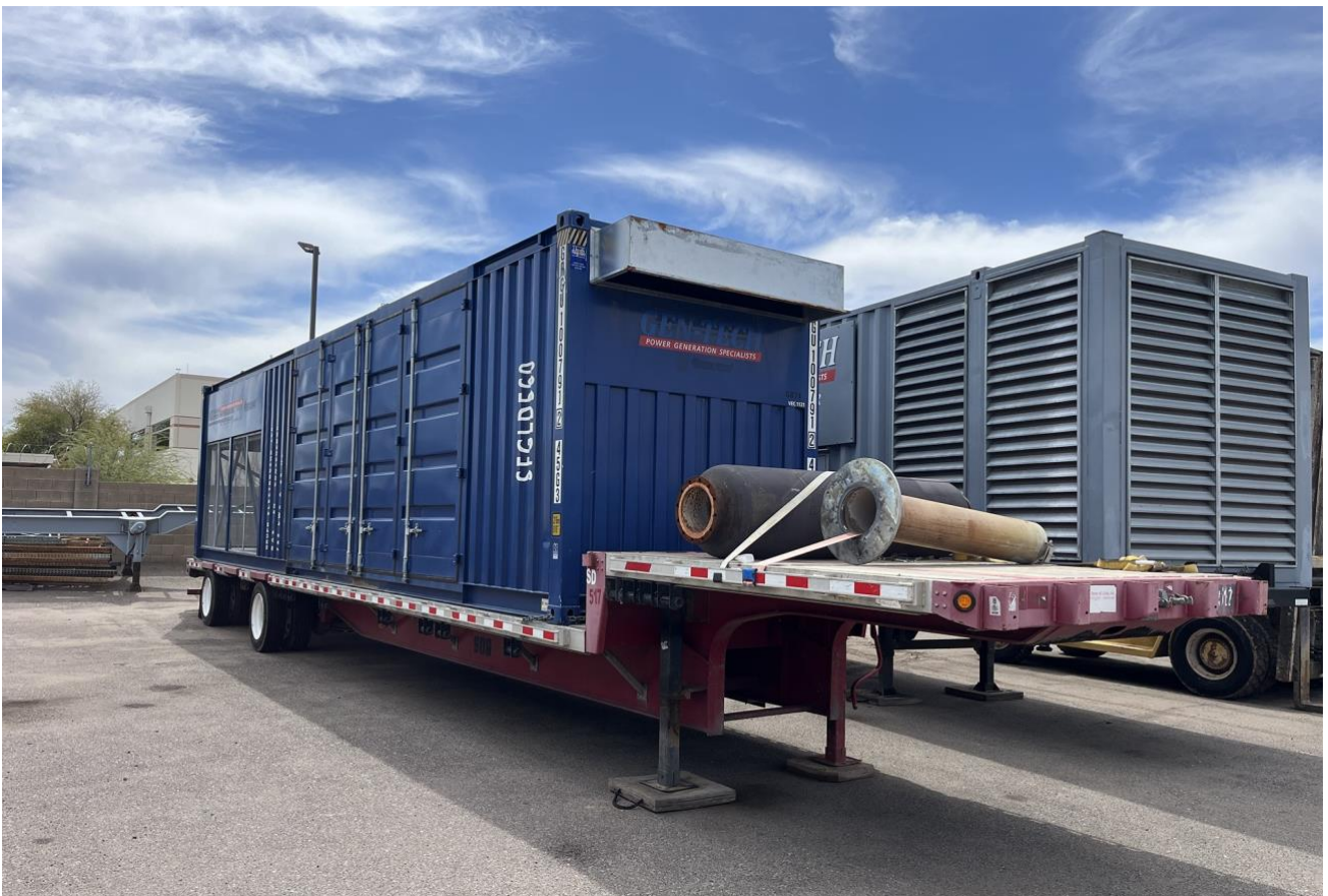
FIGURE 1: FIRST GEN-TECH GENERATOR READY FOR MOBILISATION
