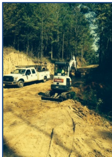
SITE CONSTRUCTION OPERATIONS PREPARE THE LOCATION FOR OIL COLLECTION & HAULAGE
