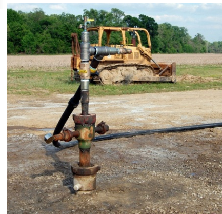
Saltwater Injection Well
