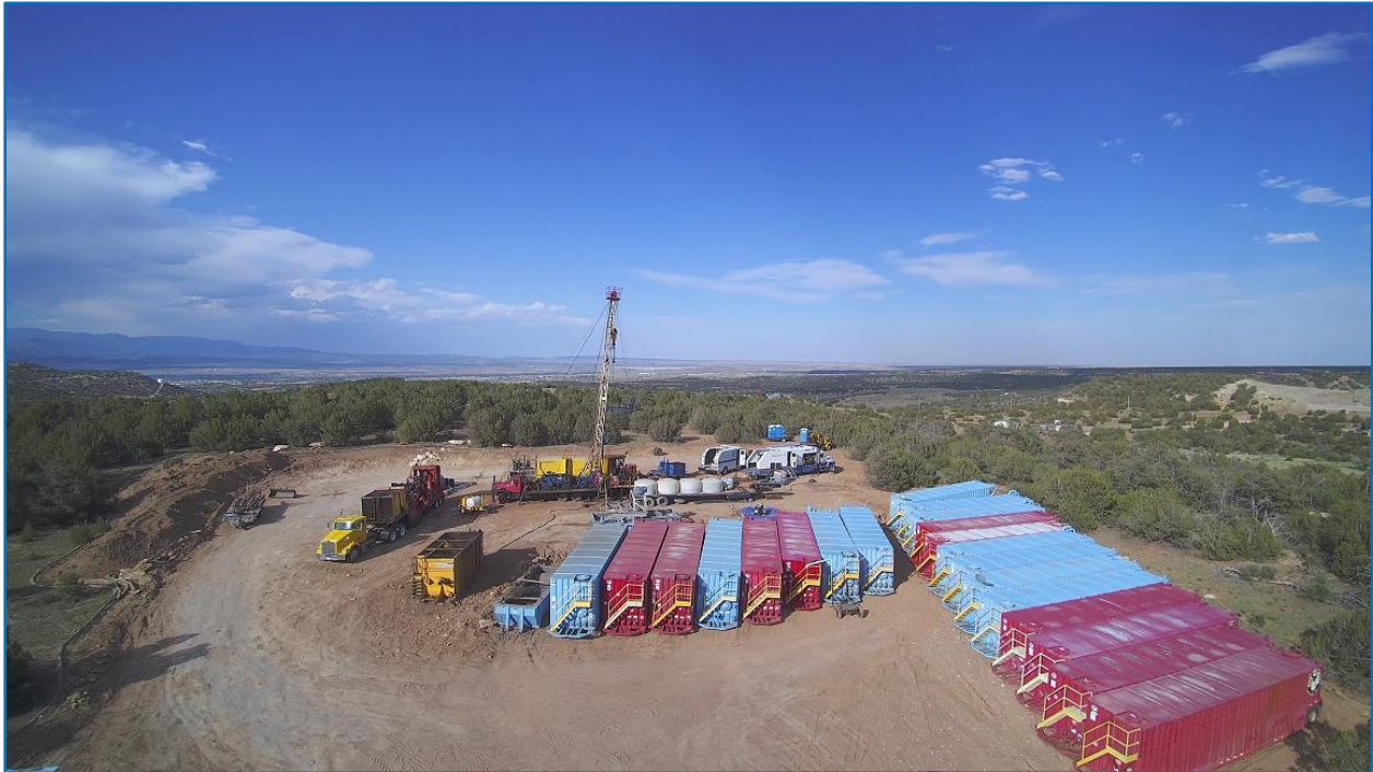
Figure 2: Completion operations on the Amerigo Vespucci #1 well.
