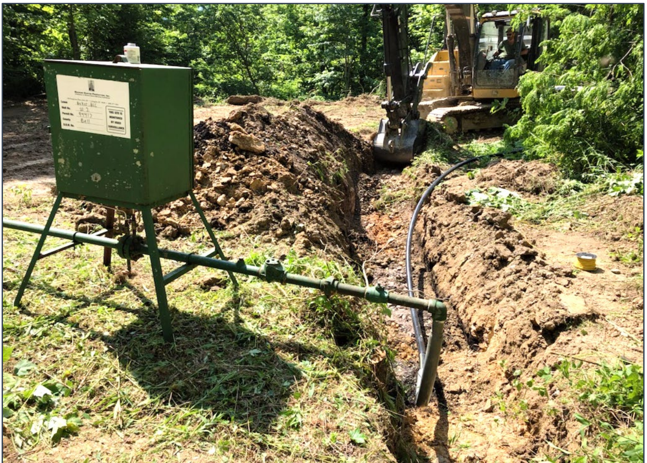
FIGURE 2: PREVIOUSLY OFFLINE GAS WELL BEING TIED BACK INTO NEWLY LAID PIPELINE
