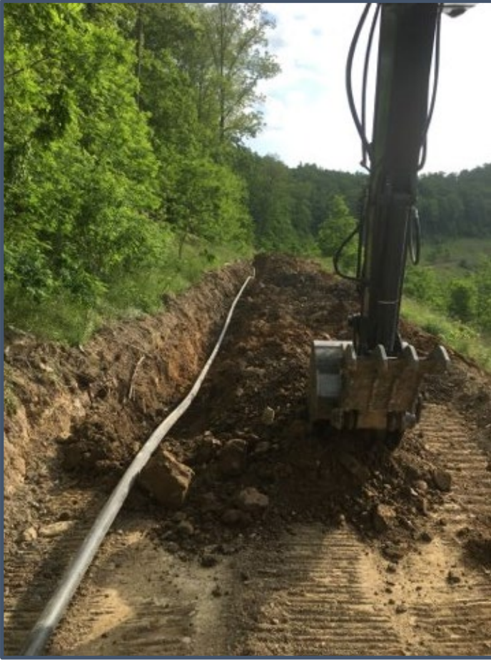
FIGURE 3: NEW 2-INCH PIPE BEING RUN AND CONNECTED
