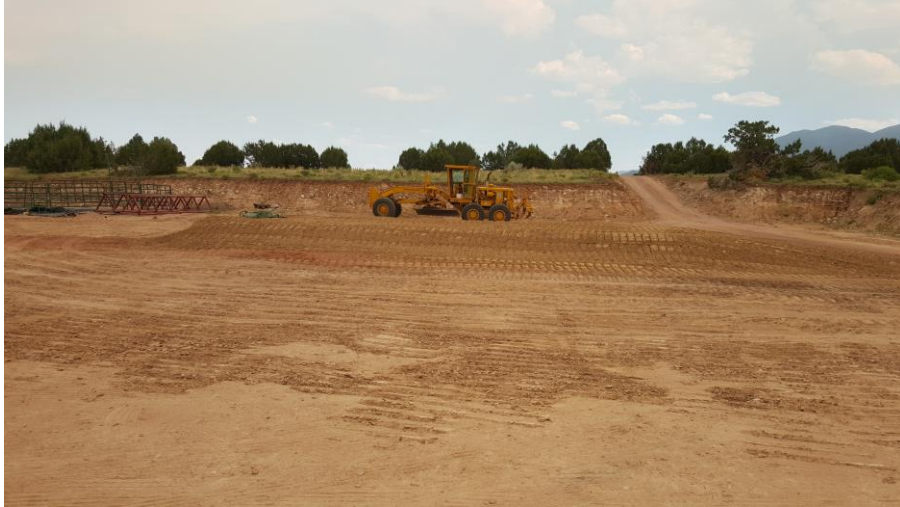
Preparing the Marco Polo well pad
