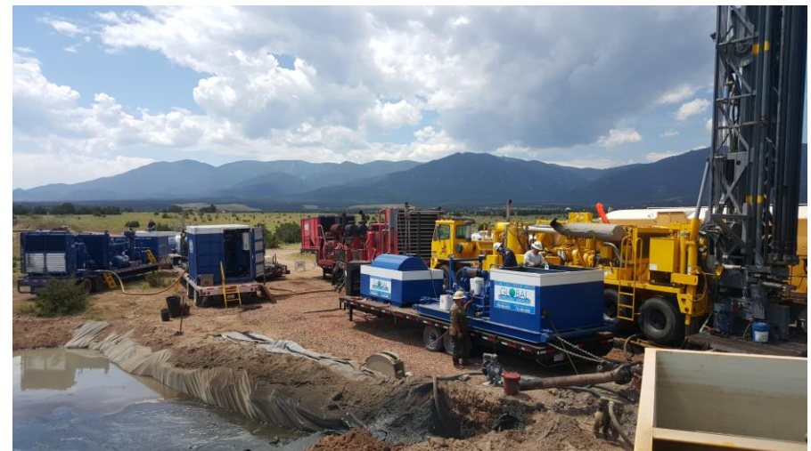
Drilling equipment layout during drilling of Magellan
