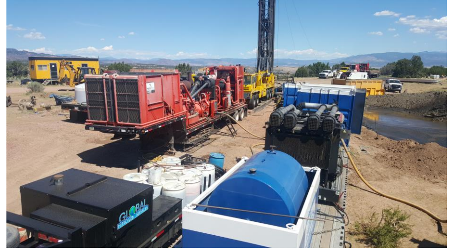
Drilling equipment layout during drilling of Magellan
