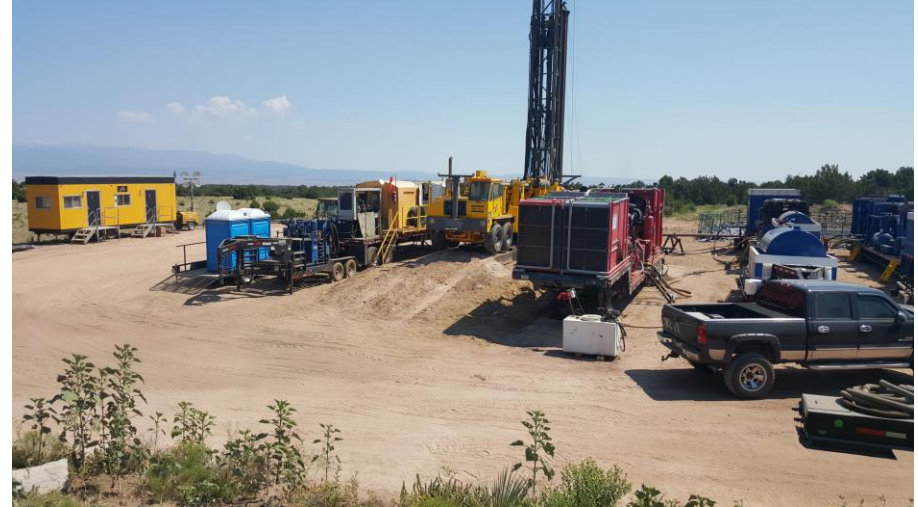
Drilling equipment mobilized in preparation for the drilling of Marco Polo
